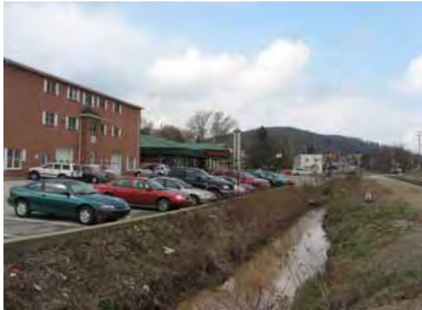
Existing Condition of Whites Run Adjacent to Development
