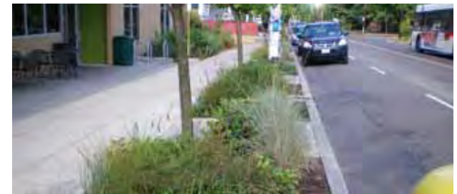
Rain gardens and inlets
