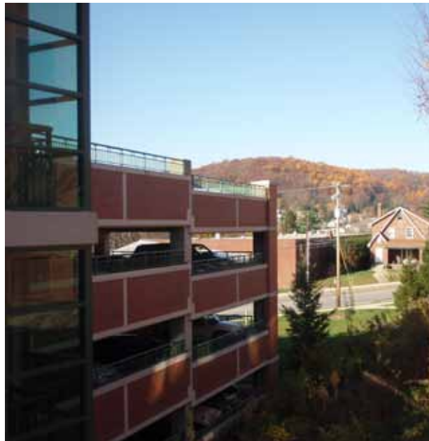
Existing parking structure
