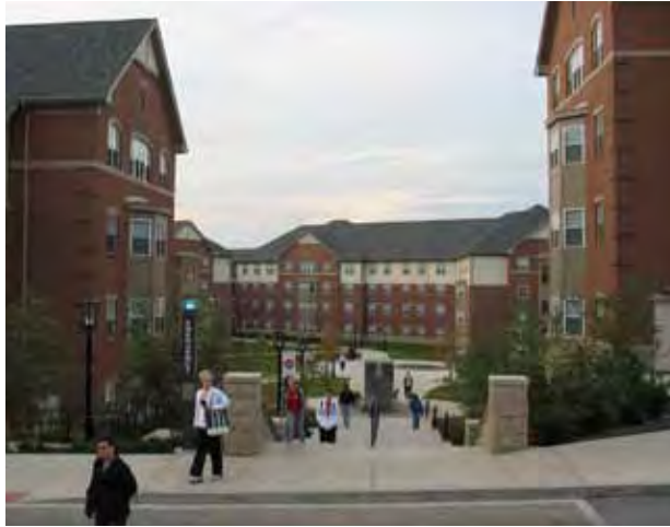
Residential Revival Suites at Grant Street
