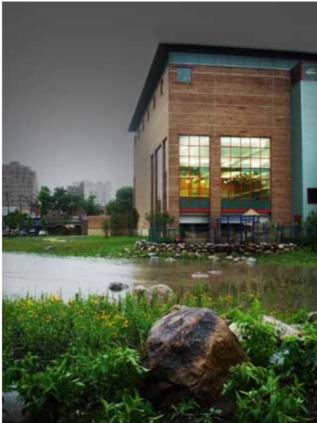
Wetland plantings and stormwater treatment
