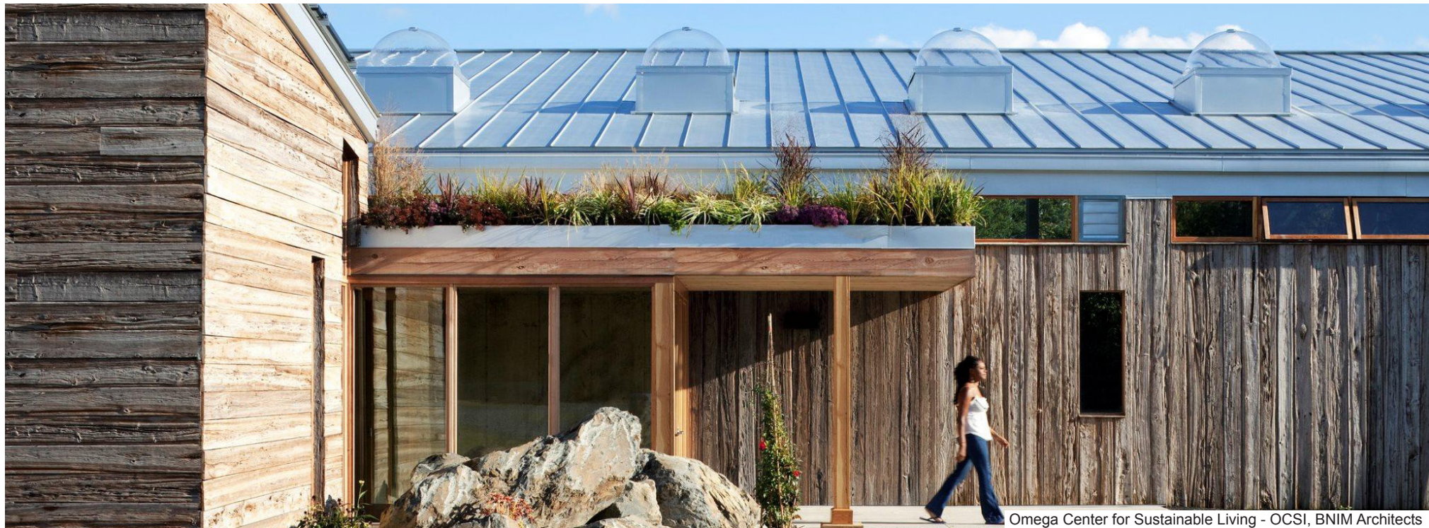
Omega Center for Sustainable Living - OCSI, BNIM Architects
