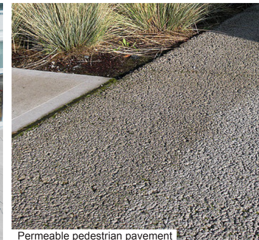
Permeable pedestrian pavement
