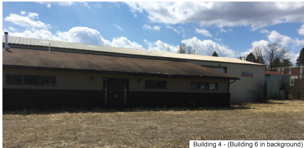
Building 4 - (Building 6 in background)
